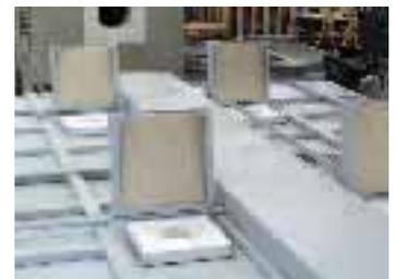
Automatically controlled vapour vent flaps
