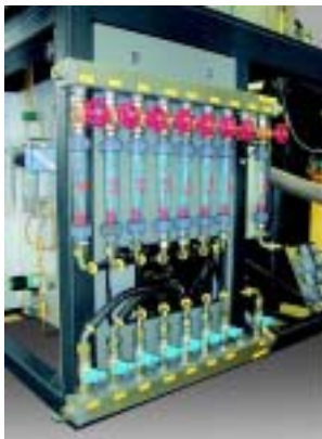
Cooling water supply
